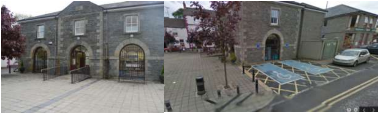
Front of the Market House (Library Building), Bailieborough, and view of the proposed site to the side of the building (disabled parking bays to be relocated).
